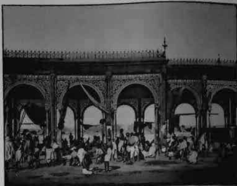
The Armenian Ghats were built in 1734 by Manick Hazare Malabar, a celebrated trader of Armenian origin. This elegant structure was one of the many contributions made by the business Armenians to develop the infrastructure and multicultural support of Calcutta as city to build.
