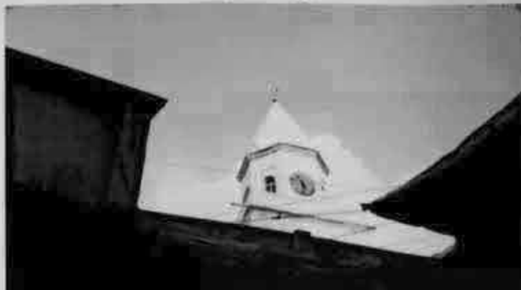
The Holy Nazareth Church is the oldest church in Kolkata. Built by Aghe Maron in 1724 after the original existing wooden structure was destroyed in a fire in 1658. Today, the Bell of the Church keeps out from a temple of stone and concrete masonry. Image: Santanu Sengupta
