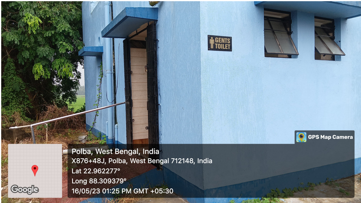
GENTS TOILET WING WITH RAMP
