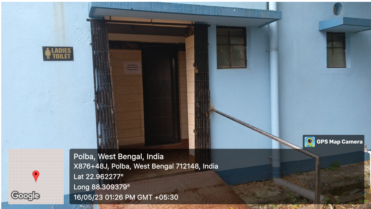
LADIES TOILET WING WITH RAMP
